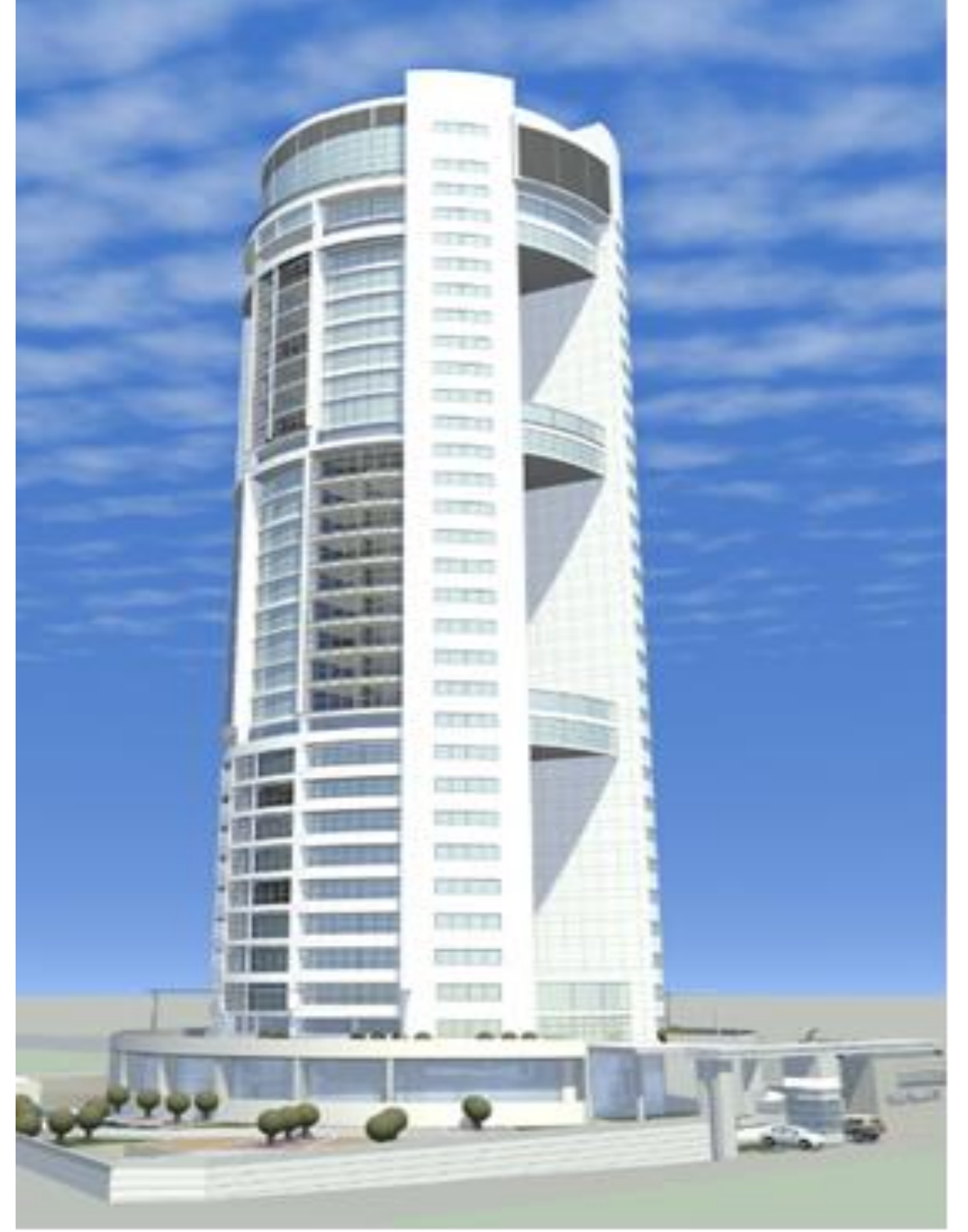
GARAGE İNŞAAT MERTER KULE - MERTER ISTANBUL (2010)
